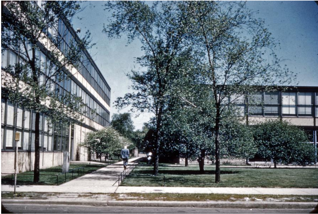
IIT Buildings and Grounds. Photographed by Mildred Mead in 1962. University of Chicago Photographic Archive, [apf2-10020], Hanna Holborn Gray Special Collections Research Center, University of Chicago Library.
